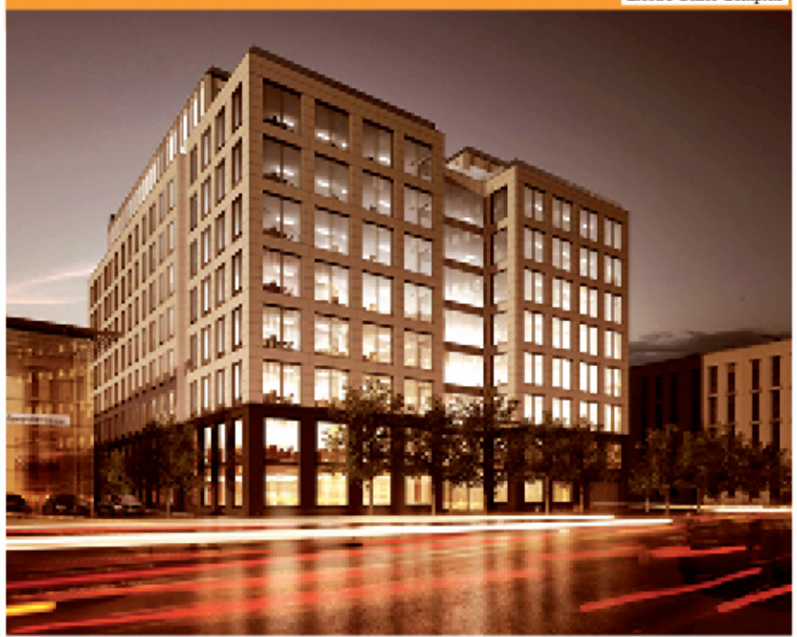
Electro Office Complex
